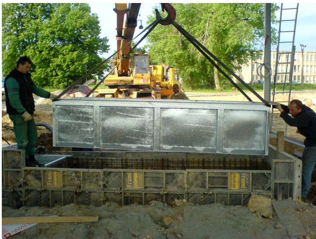
Blocker's frame settling on top of foundation plate
