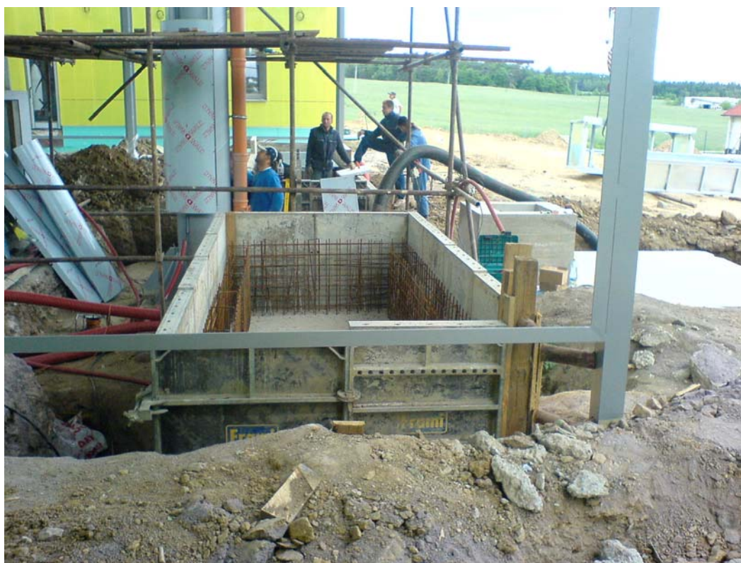
Foundation plate concreting where blocker is settled
